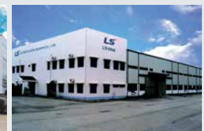
Hanoi Factory (Vietnam) MV/LV switchgear, Mold TR
