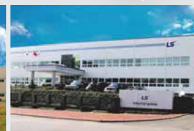
Dalian Factory (China) MV/LV switchgear, MV contactor
