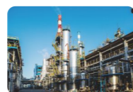
Industrial circulation system
