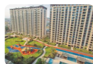
Domestic water pressurization
