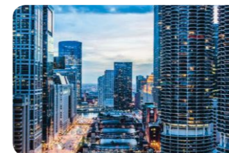
High-rise building pressurization and supply
